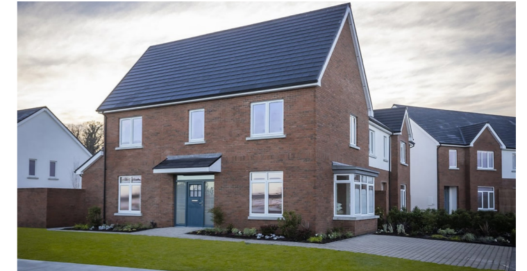
PHASE 1 HOUSING IN BELCAMP
